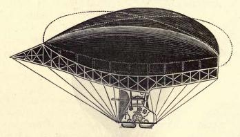
A fan or propeller is driven by treadle mechanism, and the passengers are provided with seats within a closed car. Four boats are carried below the car for supporting the apparatus should a descent be made on water.
